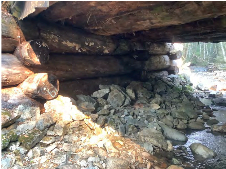
Right Bank Abutment when facing downstream
