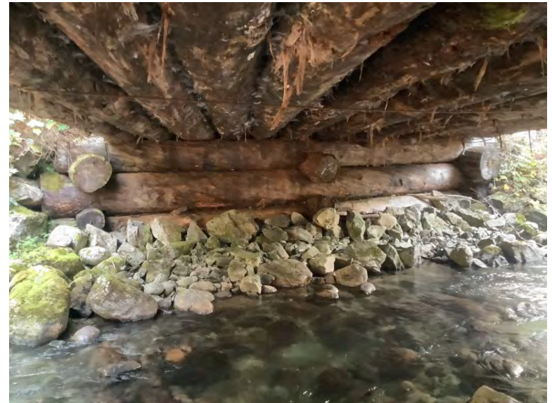
Left Bank Abutment when facing downstream
